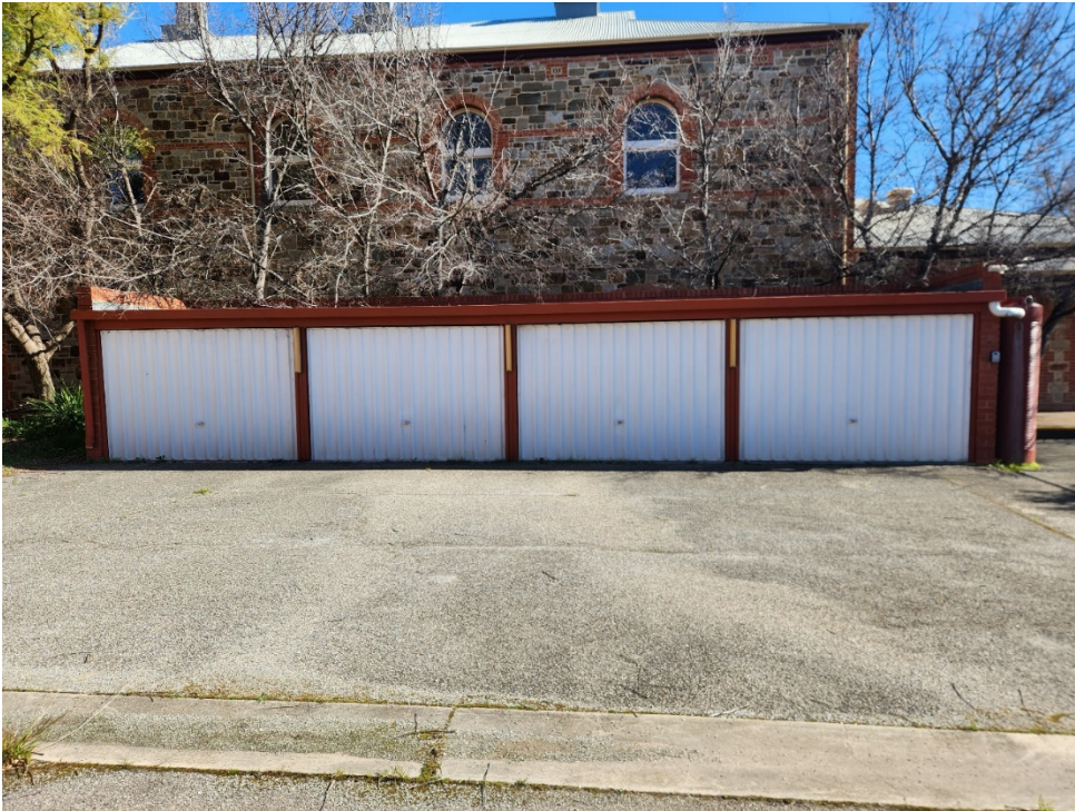
Figure 4: Storage sheds adjacent to the community centre – external view
